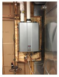
New tankless gas water heater passed inspection though inspector needed installation manual to inspect...probably never seen one before? New air filtration system also installed.
